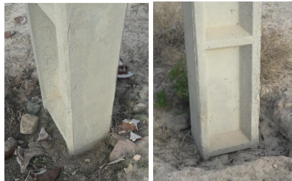
Fig. 4. No visible damage at pole anchors of Armak-Charak main (suspension insulators, soil backfill, 1994)
